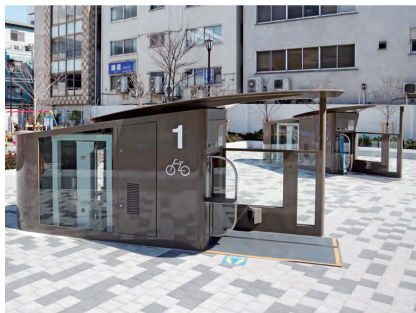
Shinbashi Station, Tokyo
